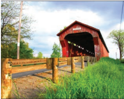
Swartz Bridge, Wyandot County, Ohio
